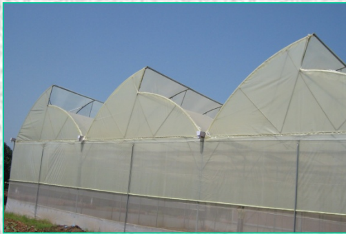
A naturally ventilated greenhouse: Screened sidewalls and roof vents
